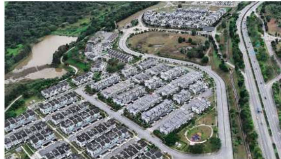
Infrastructure Works for Precinct 12
