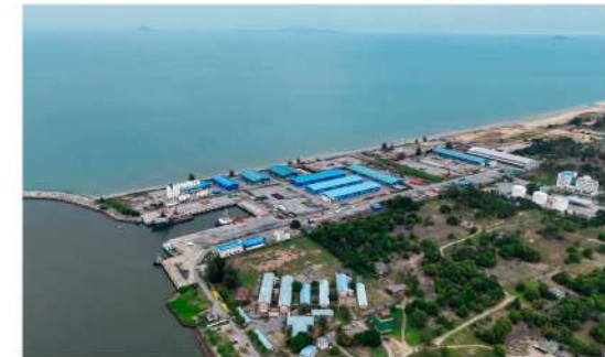
Tok Bali completed site
