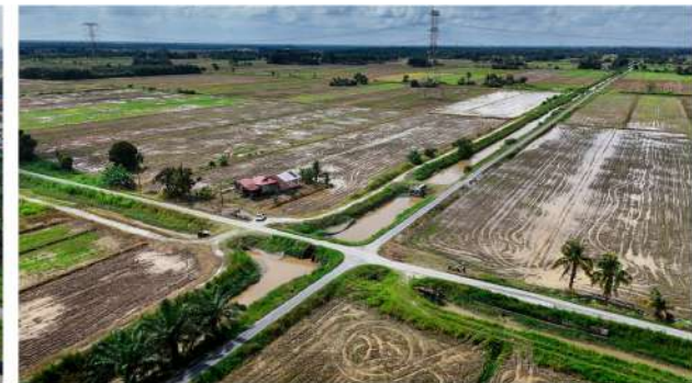
Sg Manik drainage & irrigation
