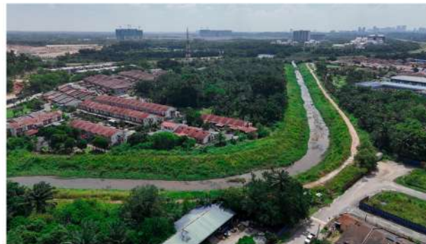
Flood barrier in Dengkil
