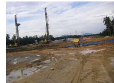
Stone column installation
